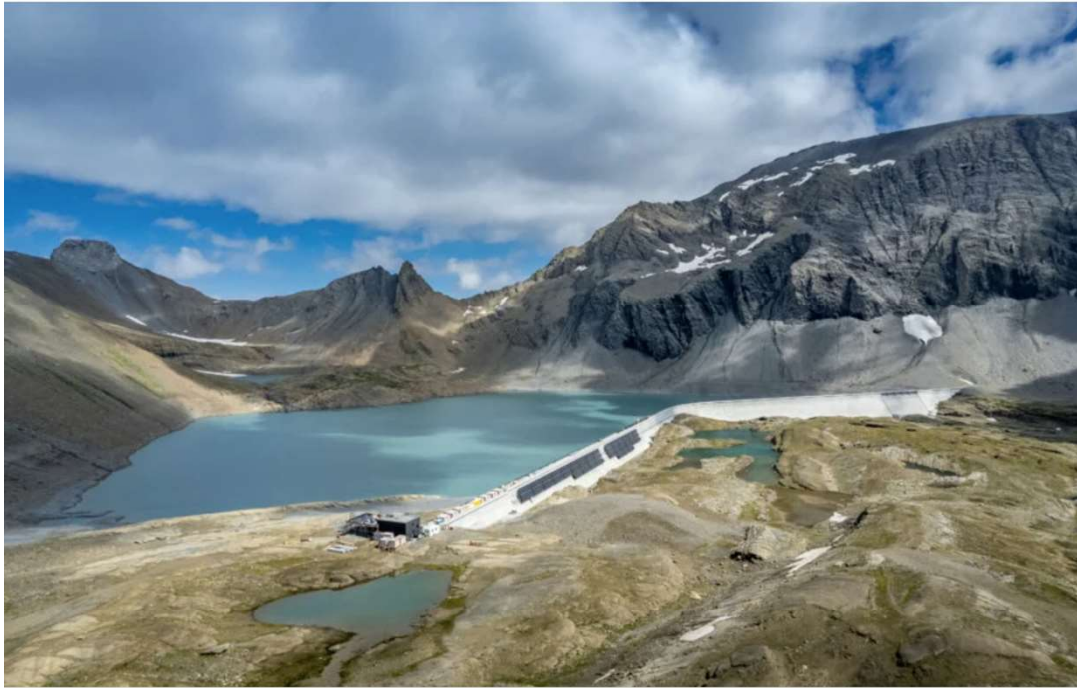
The solar plant on Muttsee dam (under construction here) reaches maximum output when snow reflects sunlight onto the cells © Axpo AG
