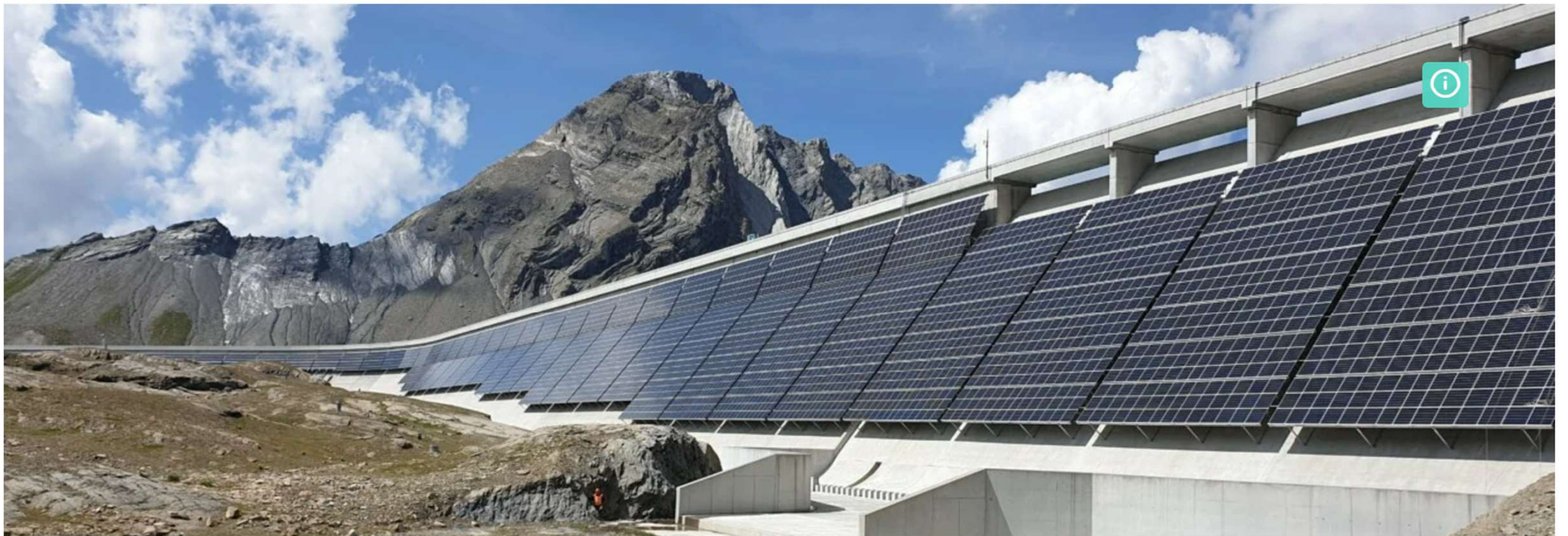
The solar plant on Muttsee dam (under construction here) reaches maximum output when snow reflects sunlight onto the cells © Axpo AG
