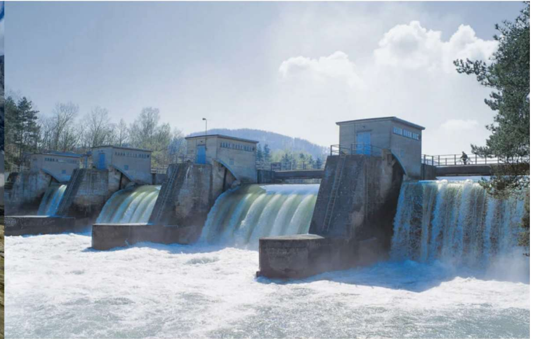
Run-of-river power plants like the one in Wildegg-Brugg meet 35 per cent of Switzerland's electricity needs but generate three-quarters of their electricity between May and October. © Axpo AG
